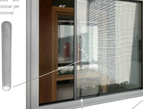
All openings are protected from unexpected ember attack through heavy-duty fly screens, which combine strong extruded frames with Stainless Steel mesh
